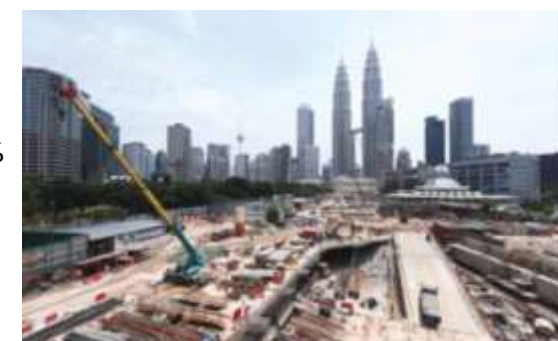
KLCC North East Car Park, Package 2 & 2A
